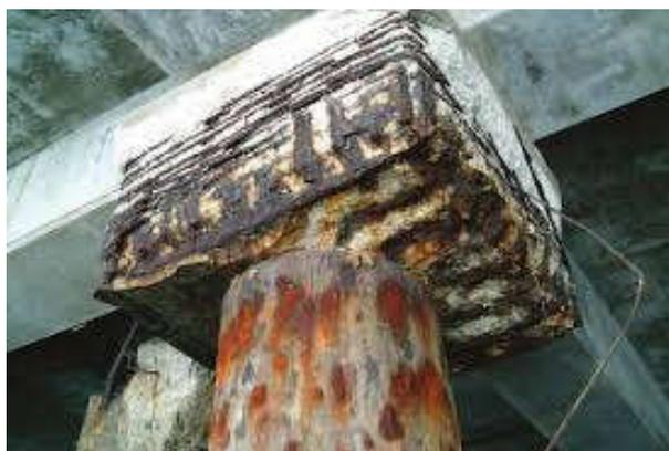
**Fig.1. Corrosion due to ingress water**
