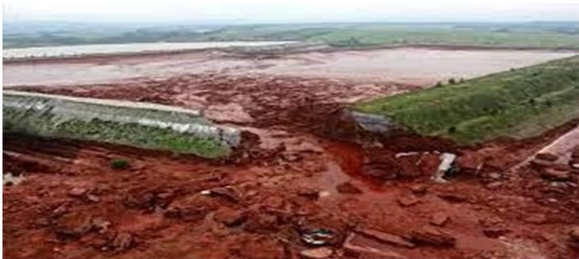
Fig.1.16. Collapse of Ajka Bauxite Tailings Dam, West Hungary, 2010 (After Evans, K, 2015)
