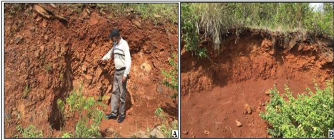
Fig. 1.11. Slope cuts sampled for Mineral Evaluation, Ainamoi Area
